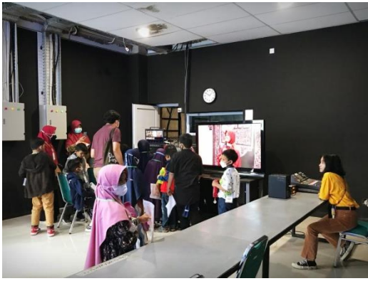
Gambar 1. Ruang kontrol utama/MCR ( master control room )
